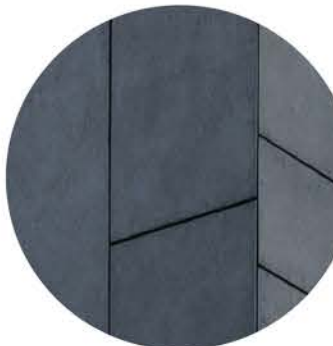
Concrete panels in the first floor
