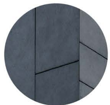
Concrete panels in the first floor
