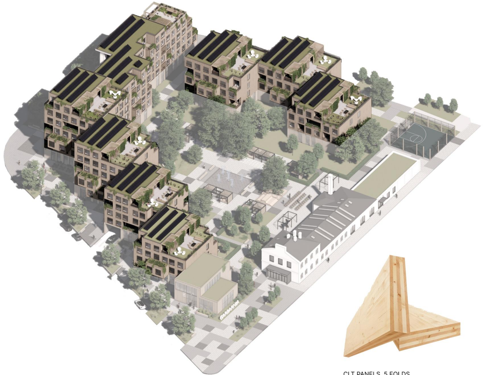
CLT PANELS, 5 FOLDS 625x prefabrication wooden modular units 2916 m 2
