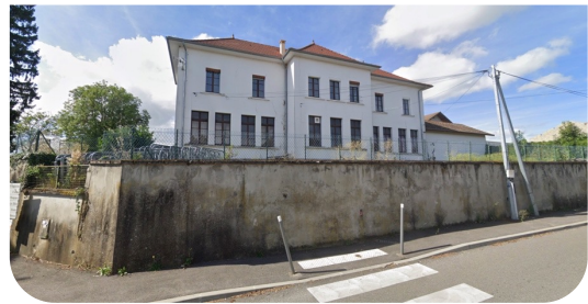
View of Old School Building in Chimilin
