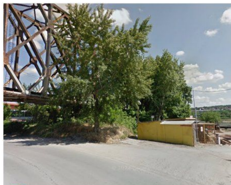
3 Infrastructure and greenery
