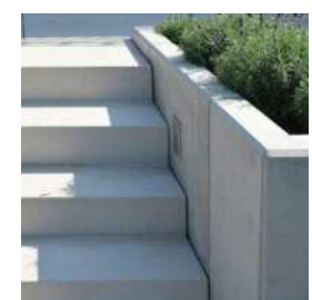
STAIRS - POLISHED CONCRETE WITH INTEGRATED LIGHTS
