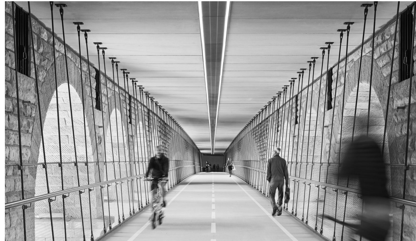
Reference : Christian Bauer suspends pedestrian and cycle path beneath Pont Adolphe, Luxembourg
