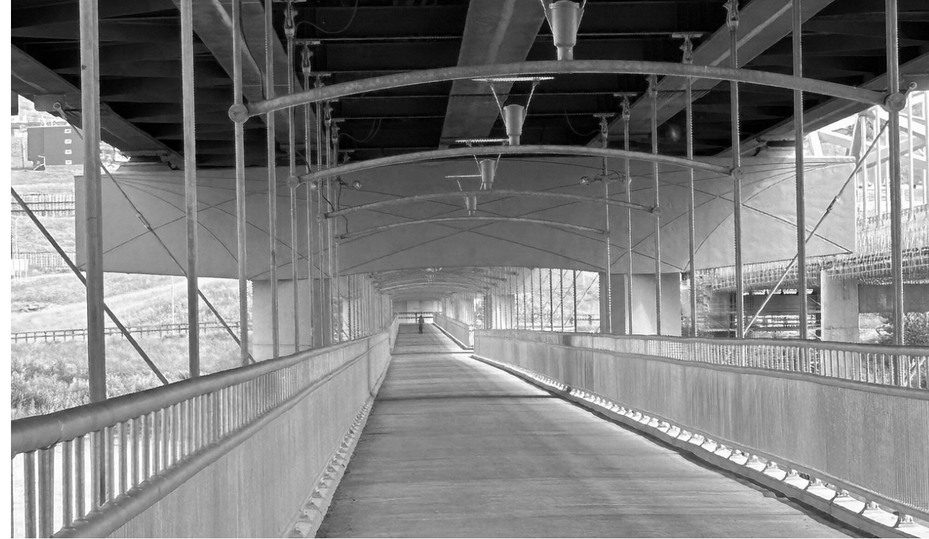
Reference : Suspended Under-Bridge Walkway Over Peace River, Canada
