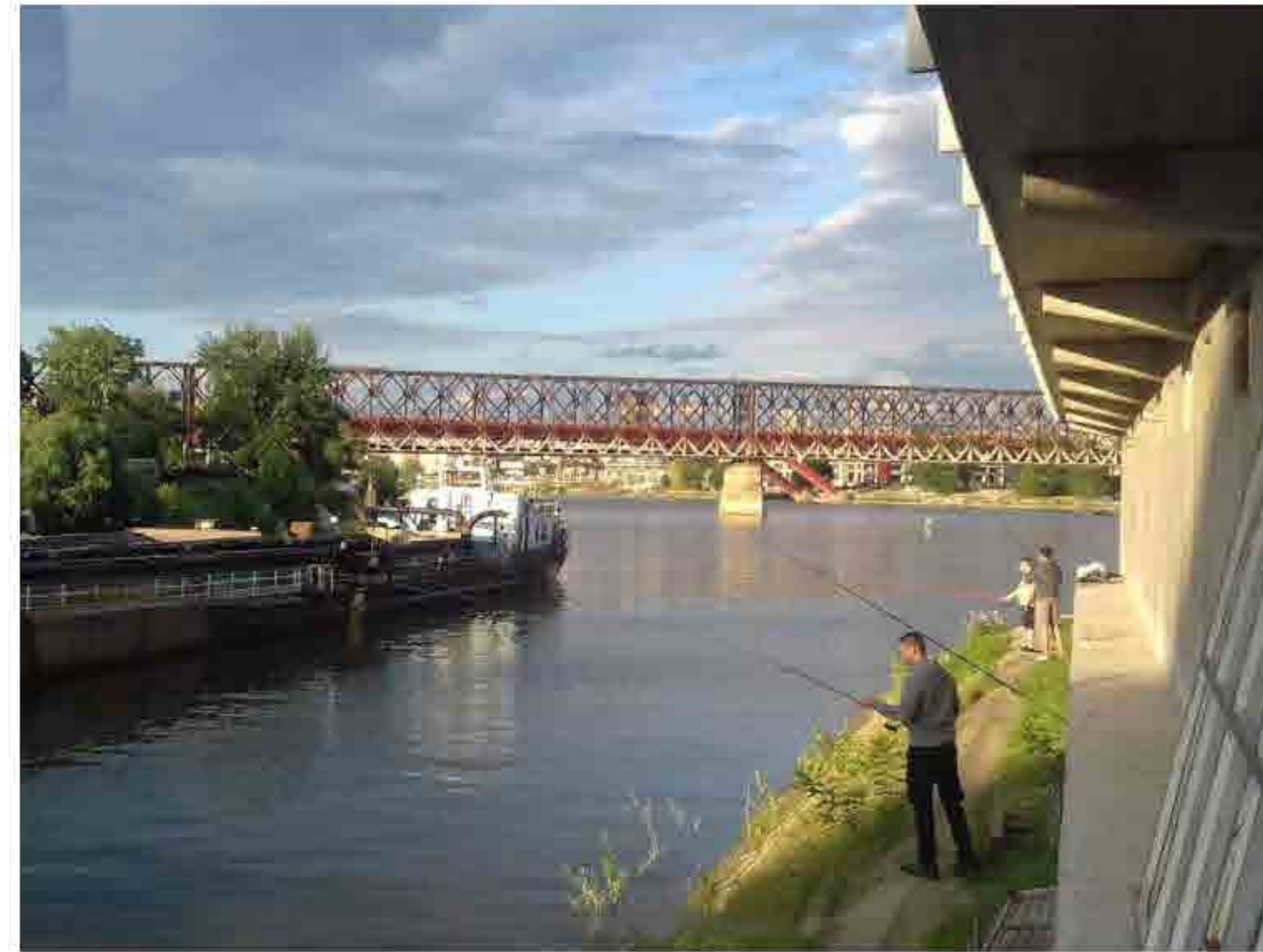
Insufficient Ecological Expression
