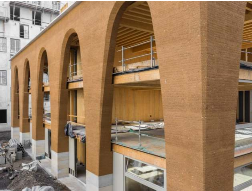
LOCAL PISÉ (RAMMED EARTH) CONSTRUCTION
