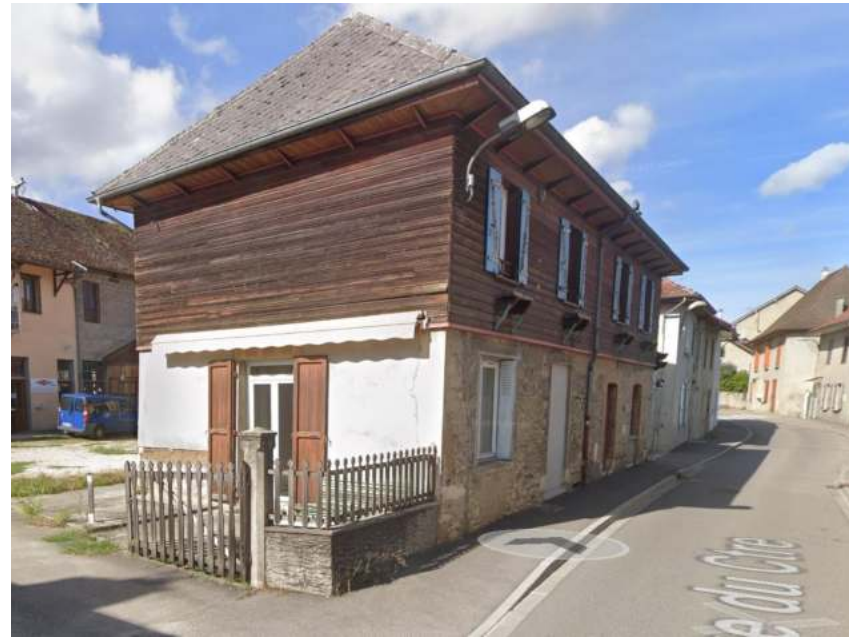
HYBRID MASONRY AND WOOD
