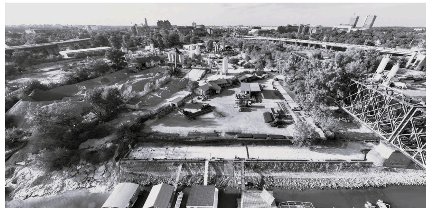
Existing site conditions
